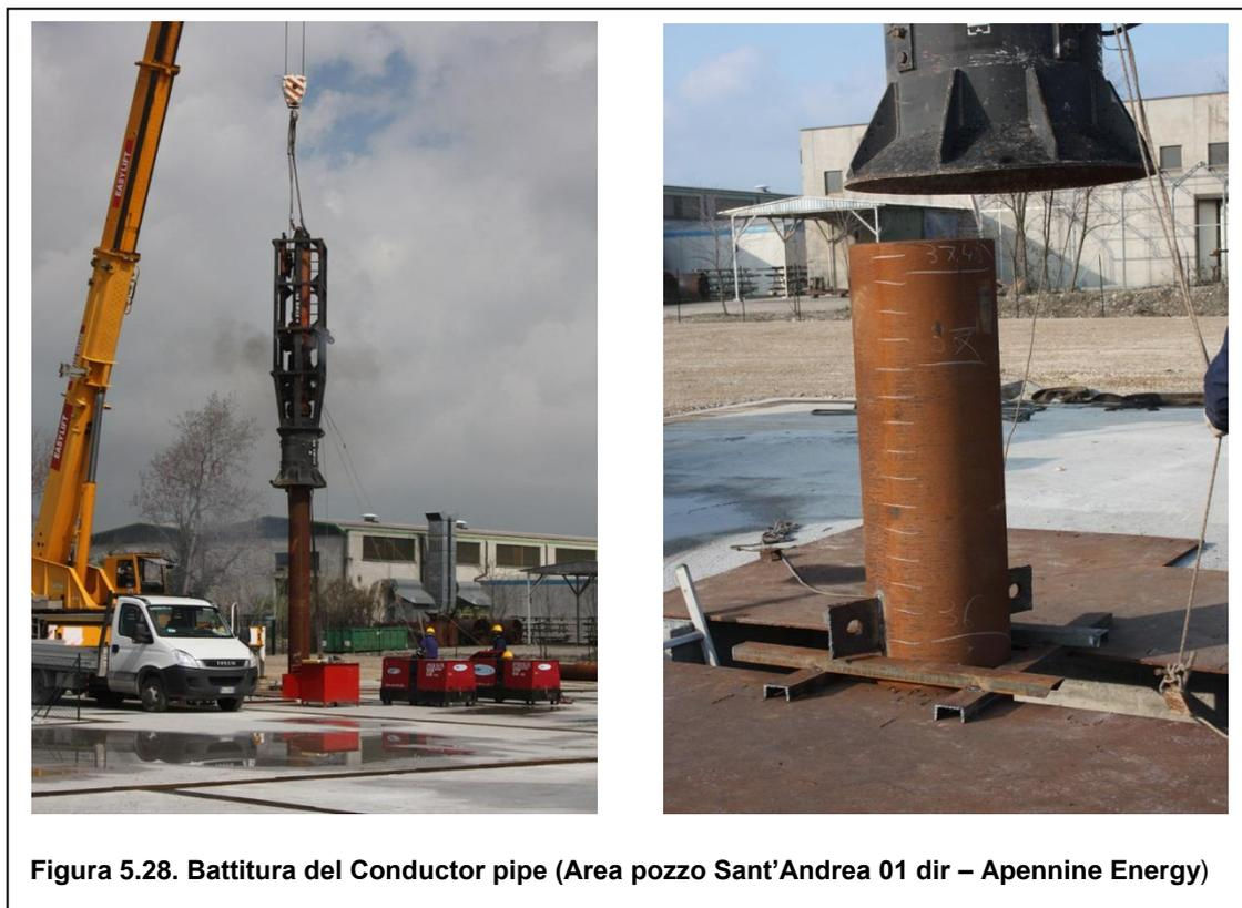
**Figura 5.28. Battitura del Conductor pipe (Area pozzo Sant'Andrea 01 dir – Apennine Energy)**
