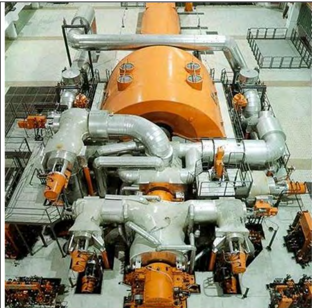
Figure 2.17: Steam turbine of a coal-fired power plant
