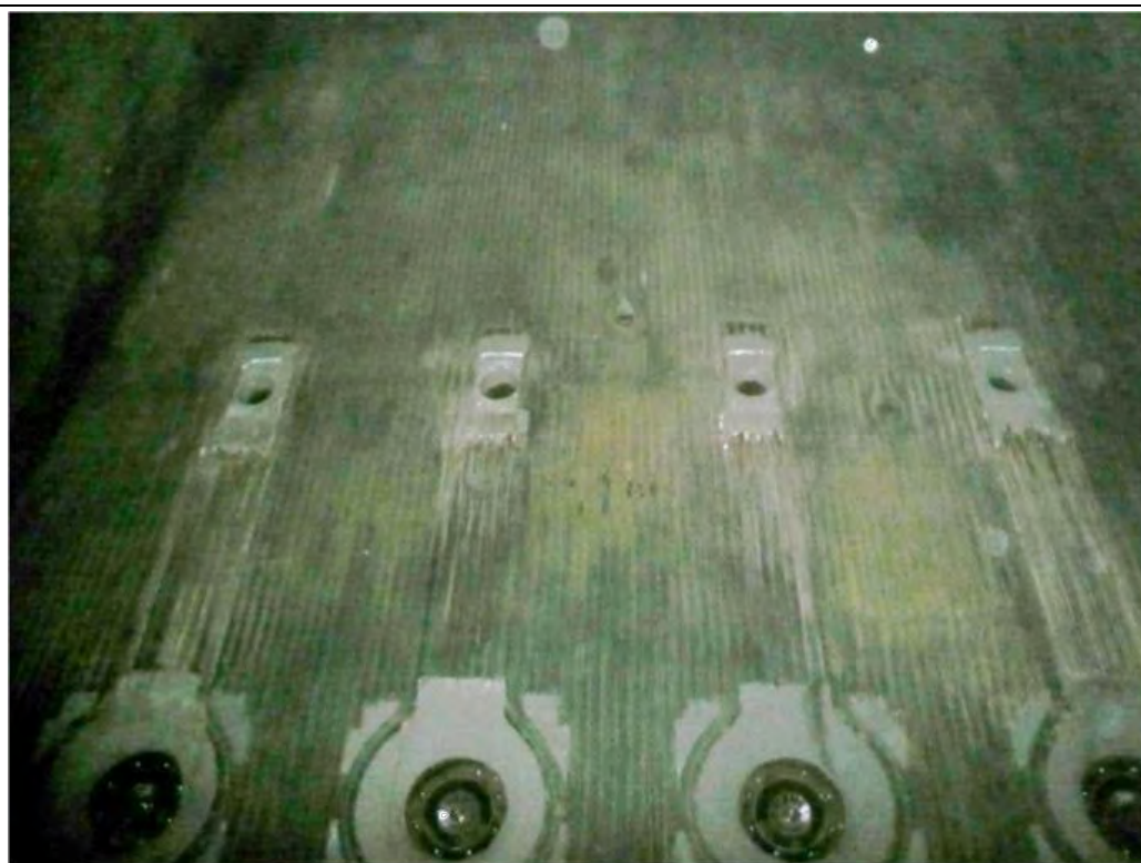
Figure 8.9: Overfire air technique retrofitted in a boiler at a chemical installation
