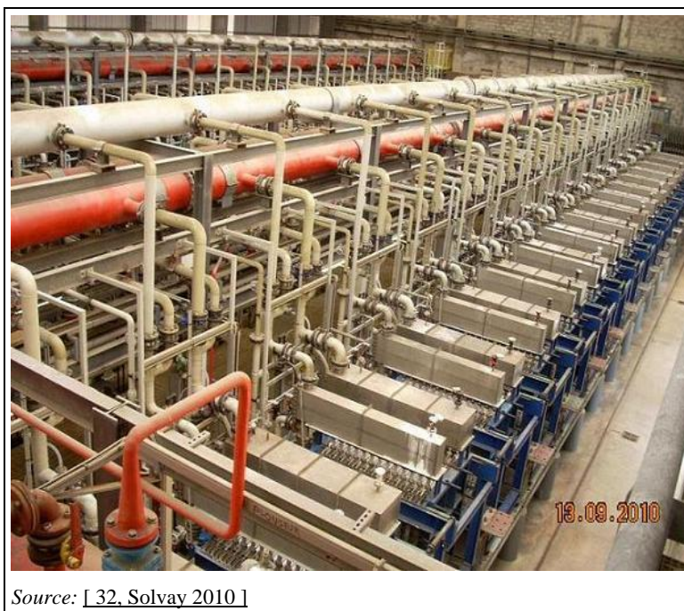
Figure 2.11: View of a membrane cell room equipped with monopolar electrolyzers
